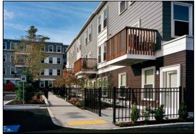
Spencer Green is one of several major residential developments that have replaced industrial and institutional uses on Spencer Avenue. Spencer Green is a $15m, 48-unit affordable rental development of Chelsea Neighborhood Developers.
