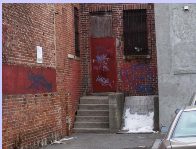
The Rear of Luther Place
