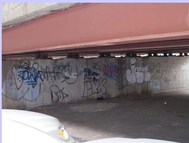
Under the Bridge near The Williams School
